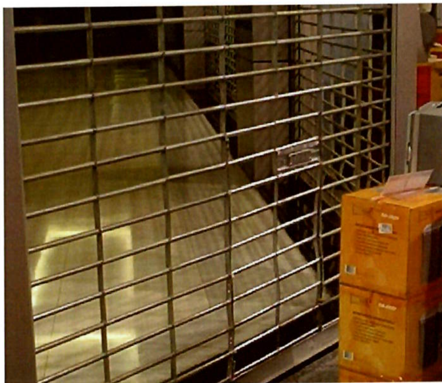
Fig. 30 – portinhola vertical retrátil dim(1,10 x 0,62 )m.
